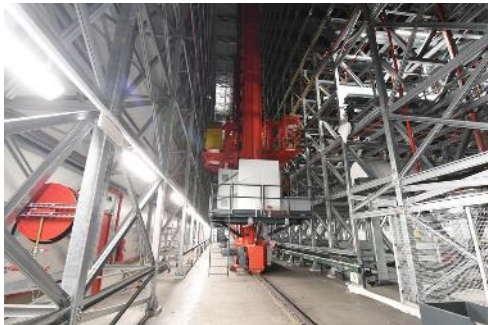
Automatic Reel Storage 10.000 T
